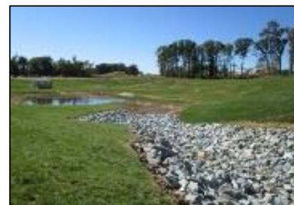
Figure 1 – Detention Pond Using BMPs
